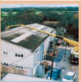
Mechanical plant being used to inspect a fragile/brittle roof.
