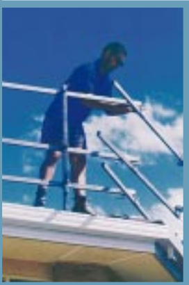
One of many roof edge guardrail systems available.
