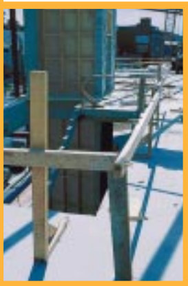
Isolating a fall hazard by barricading off a floor penetration.
